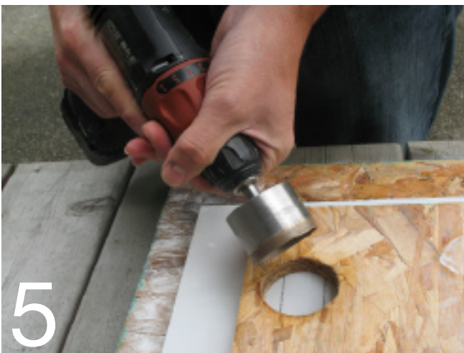
Drill on a stable surface
