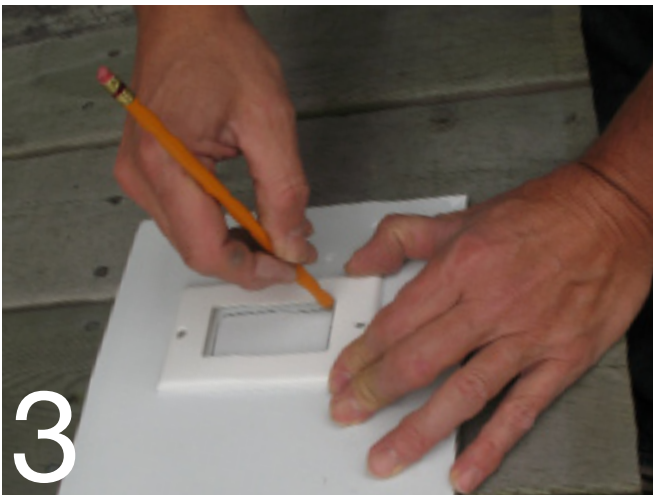
Mark the area you will be drilling through
