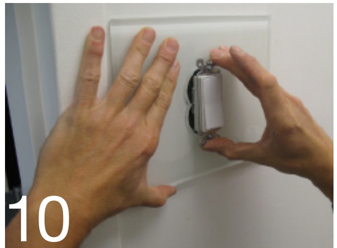
10 Install tile and receptacle
