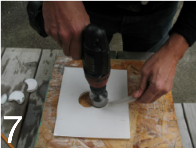
7 Superimpose a second hole to create an opening large enough to cover the recep-
